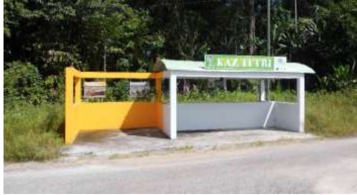
Photo 1 : Kaz Ti'Tri "MIMOSA" (zone ENC/DV + zone BACS)
